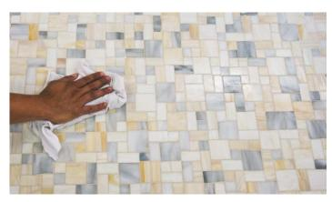
**Step 11** For final removal of grout haze, polish with a clean, soft, white cloth.
