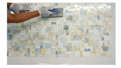
**Step 5** To achieve the flattest possible surface, lightly tap the sheets using light pressure with a grout float or a wooden beating block and a finish hammer. To unify sheet transitions, tap from one sheet to the next.
