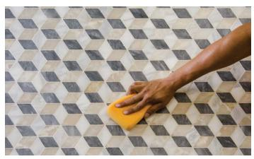
**Step 9** Allow grout to set until firm and smooth finish with a damp sponge. After approximately 2 hours, remove grout haze with a lightly damp sponge.
