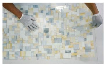
**Step 4** Apply mosaic sheets to the thinset setting bed, tape side towards you, with light, even pressure. When joining sheets, be certain to adjust sheets so that grout lines are uniform. Periodically, check thinset for skinning (slight drying). If skinning occurs, remove thinset and reapply.
