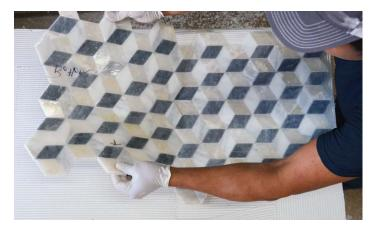
**Step 3** Apply mosaic sheets to the thinset setting bed, tape side toward you, with light, even pressure. Periodically, check thinset for skinning (slight drying). If skinning occurs, remove thinset and reapply.
