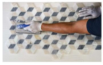
**Step 4** To achieve the flattest possible surface, lightly tap the sheets using light pressure with a grout float or a wooden beating block and a finish hammer. To unify sheet transitions, tap from one sheet to the next.
