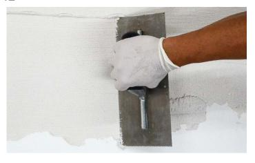
**Step 2** To establish the proper depth of the setting bed, use a  $\%_6$ " x %" v-notch trowel to apply additional thinset and comb full notches in one direction.
