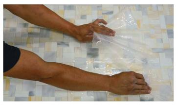
**Step 6** After 24 hours of cure time, peel the tape from the tile starting from the corner. Use an angled downward movement.
