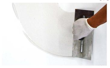
$\textbf{Step 1} \ \, \textbf{To initiate the bond coat, use the flat side of a trowel and firmly apply thinset to the substrate. }$
