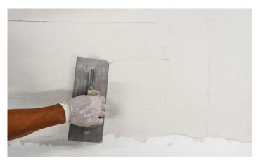
**Step 3** Use the flat side of the trowel to flatten the notches and achieve a smooth, consistent thinset setting bed.
